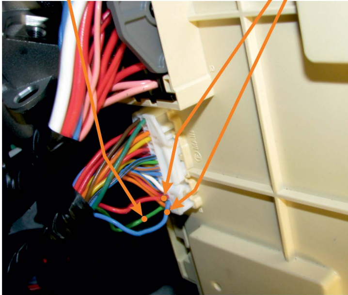
JUNCTION BOX (REAR)
